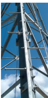
Welded Sections used on sections #13-21
